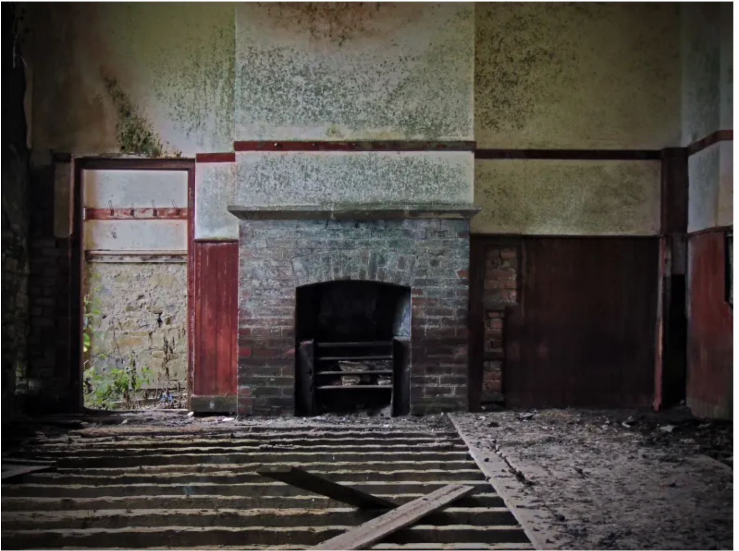
Drumreilly National School Co. Leitrim 1897
