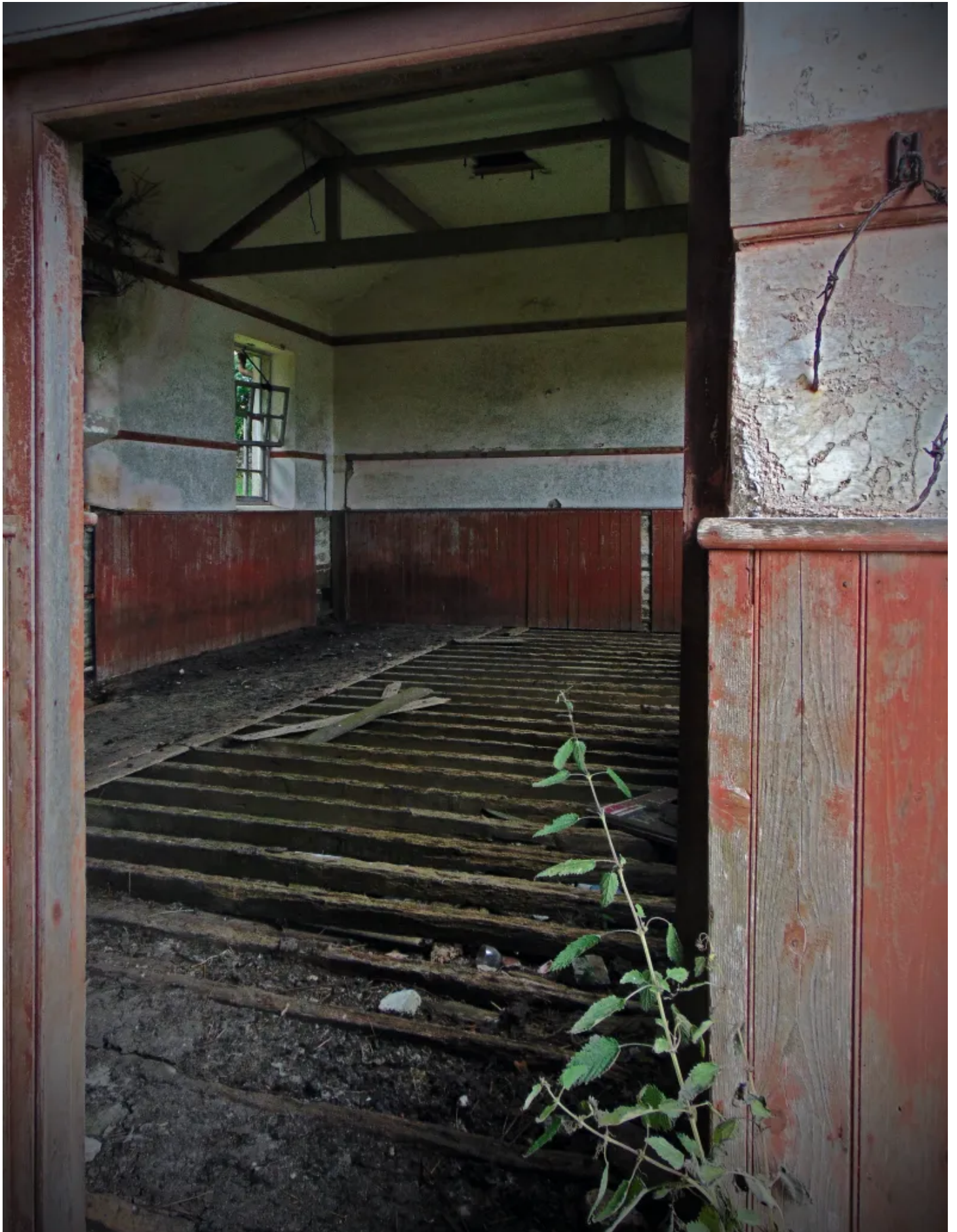
Drumreilly National School Co. Leitrim 1897
